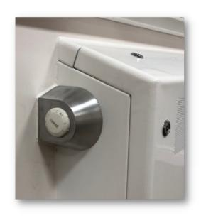
You may question the small holes around the perimeter of the valve, and you could be forgiven for thinking that these present a ligature risk. However, they have been cut in a zig-zag pattern, making it virtually impossible for a small cord to be threaded through.
